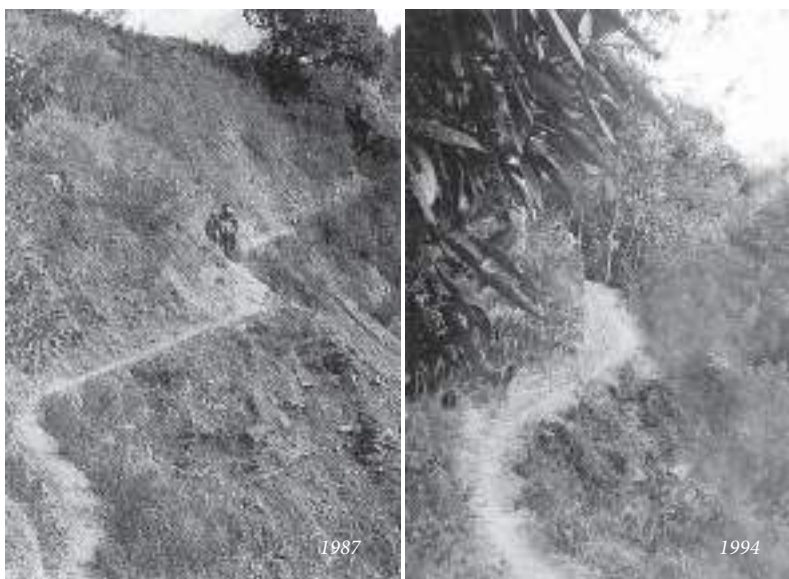
Picture 6.1: Before and after pictures of a landslide that was stabilised by managing runoff at Bhainse village, Bhattedanda, Lalitpur
