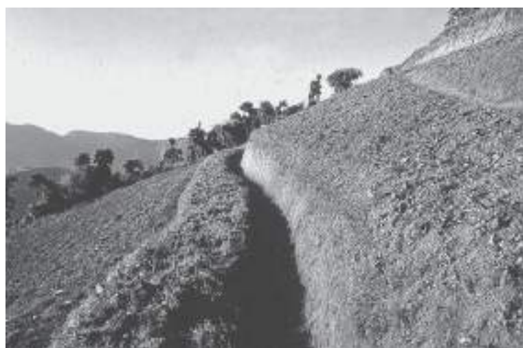
Picture 5.3: Farms with channels to divert runoff at Dalchoki, Lalitpur (1990)
