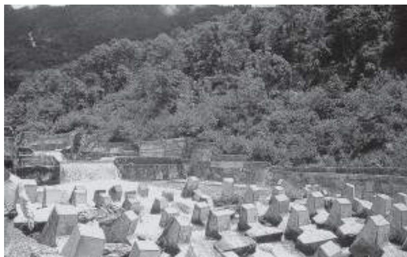
Picture 4.5: River training works at Charnawati in Dolakha District after it was damaged in 1987 by floods (1994)
