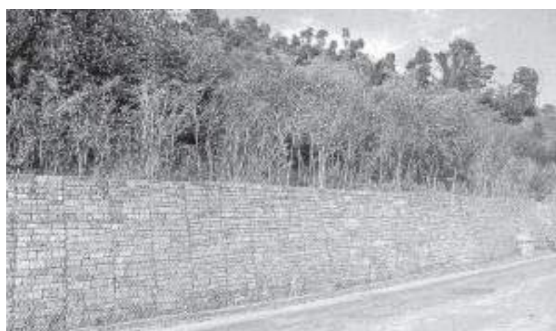
Picture 4.6: Stabilised landslide at Km 69 in Arniko Highway, Sindhupalchok (1994)
