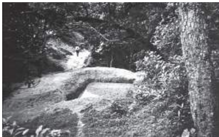
Picture 5.5b: A pond built to stabilise gullies at Bishwaroop, Pashupati, Kathmandu (1991)
