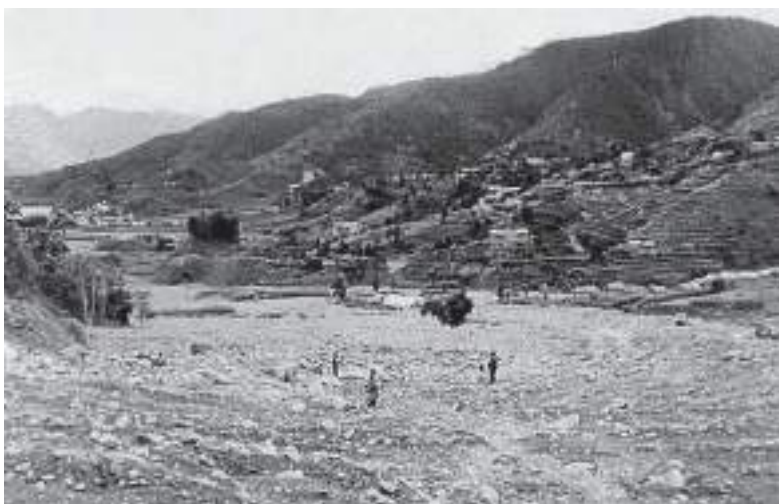
Picture 4.1a: Farms damaged by cloudburst of 1993 in Palung valley, Makawanpur (1994)
