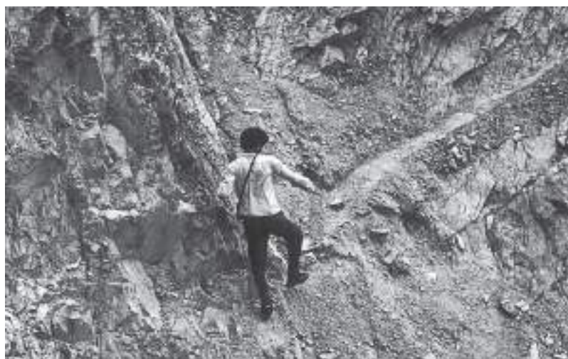
Picture 2.3: Landslide at Bukhel, Lalitpur (1991)
