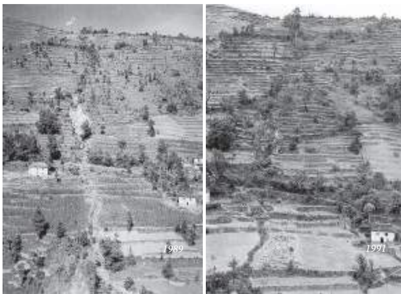
Picture 6.2: Before and after pictures of a gully stabilised by managing runoff at Bhardeo village, Lalitpur
