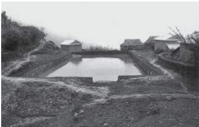
Picture 5.4: Revived pond to catch runoff at Dalchoki, Lalitpur (1990)
