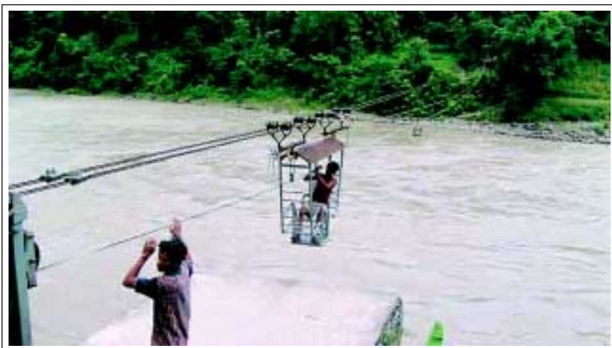
■ Tar pul in operation over the Trisuli River
