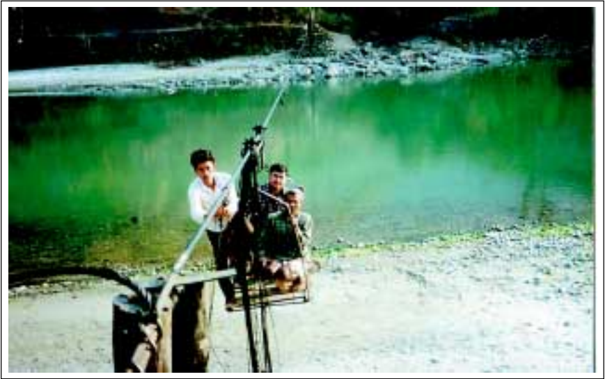
■ A ghirling consisting of a steel cable box and pulley
