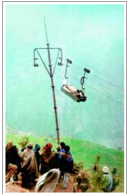
■ Ropeway in operation
