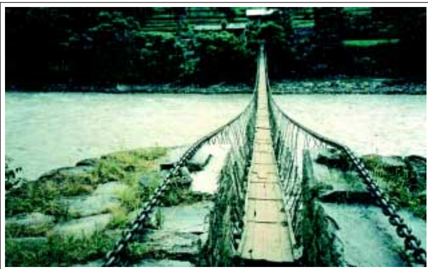
■ Suspension bridge built with chains in Baglung District
