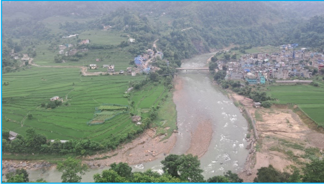
Figure 10 Flood vulnerable terraces
